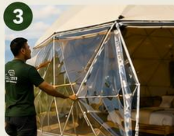
Install new window panel
